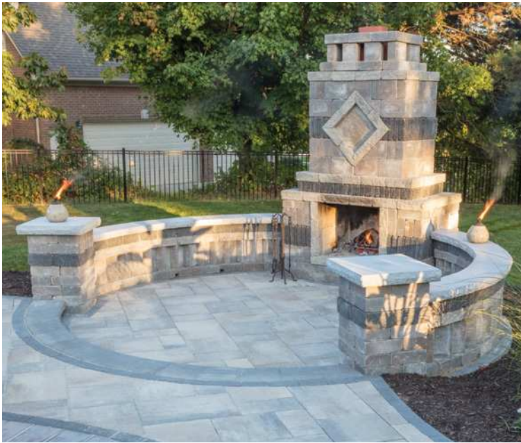
Wall, Pillars & Fireplace: Laredo, Chartan with Onyx accent Slabs: Rialto 60mm, Champagne
